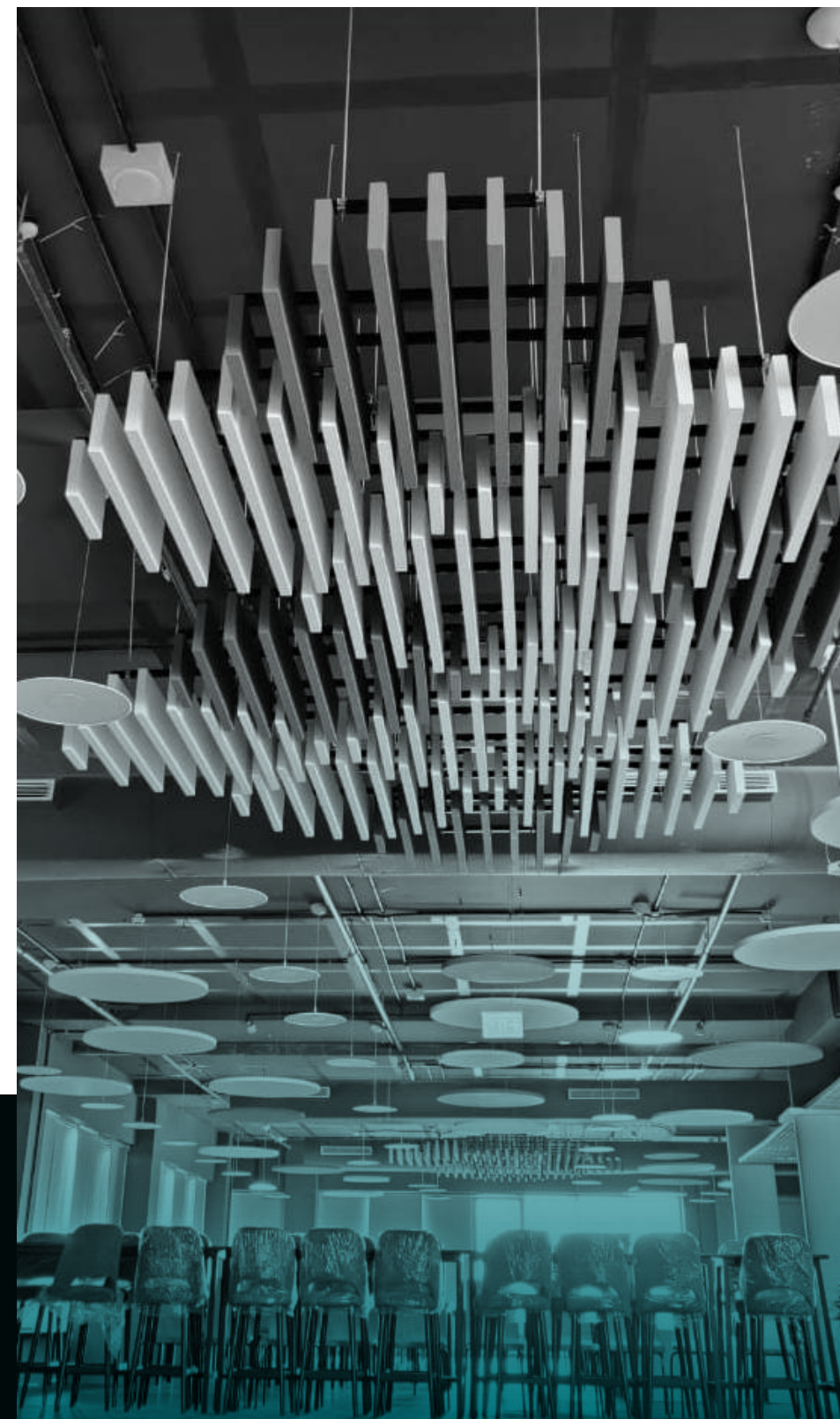
Civil & Interior Works
